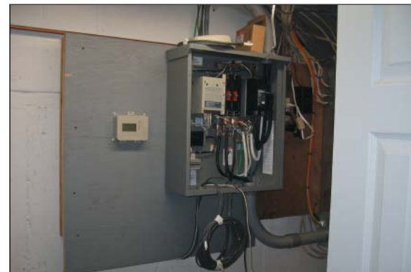
The transfer switch and the digital display being installed.
