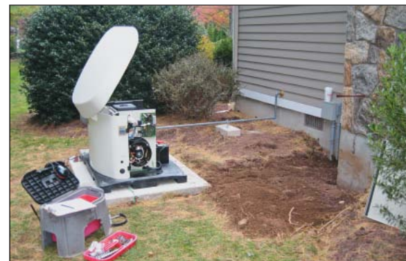
The RS20A being configured; the gas line has been connected. Piping can be installed under or above ground, depending on local codes.
